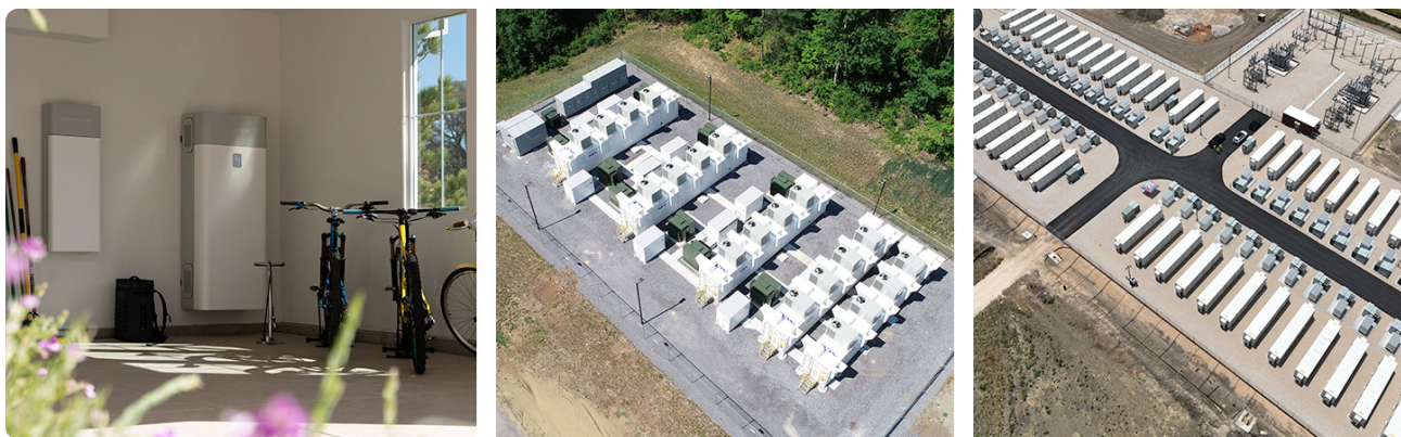
BESS at various scales: A residential on-site BESS, a small off-site BESS with 20 MW in New York, and a large off-site BESS with 100 MW in Texas. (Photos: SunPower; Key Capture Energy)
